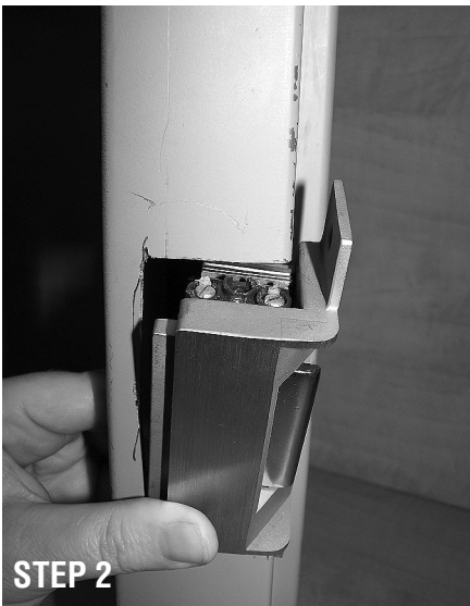
Strike Position: Rotate the strike into the frame. Note that the strike is angled slightly forward to clear the Pry-Guard.
