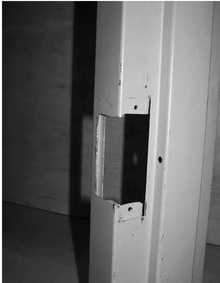
Frame Preparation: Should the frame not be cut out for the 1814 Series, follow the directions provided on page 2.
