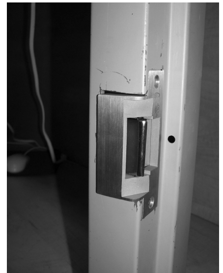
Ready to Secure: The strike is now in position ready to be secured by the two (2) 12-24 mounting screws.
