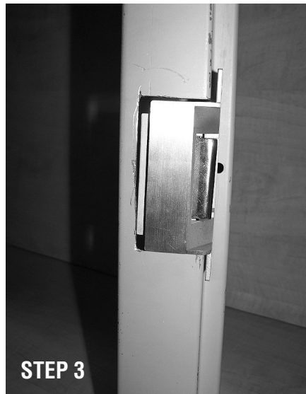
Final Push: Push the strike into the frame. The pry-guard should be behind the front lip of the frame.
