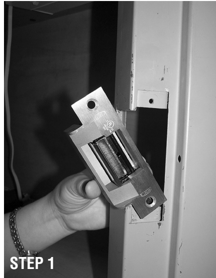
Initial Position: Place the strike as shown with the mounting tab located between the face plate and the insert.
