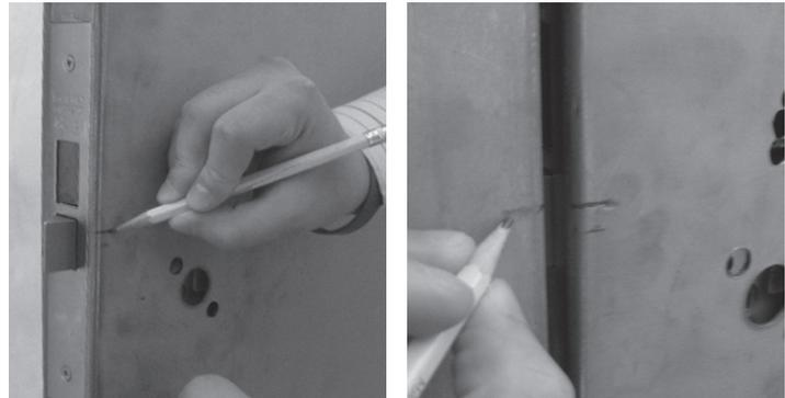
**2.** Horizontally align the proper Template Lock Centerline with the Lock Body Centerline marked on the frame. Peel adhesive backing and paste the folded template square to the frame.
