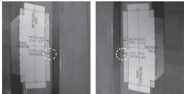
**3.** Carefully cut the frame inside the un-shaded area marked on the template. Follow Mounting Tab Installation Instructions.
