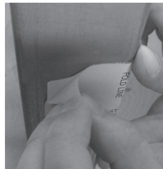
3. Carefully cut the frame inside the un-shaded area marked on the template. Install strike per installation instructions ISDYL1921/23
