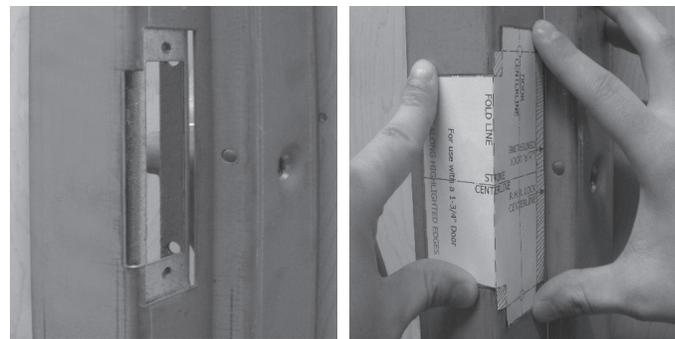
2. Peel adhesive backing and paste the folded template square to the frame.
